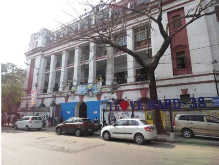
Old Building (22.5810230° N and 88.3701490° E)
