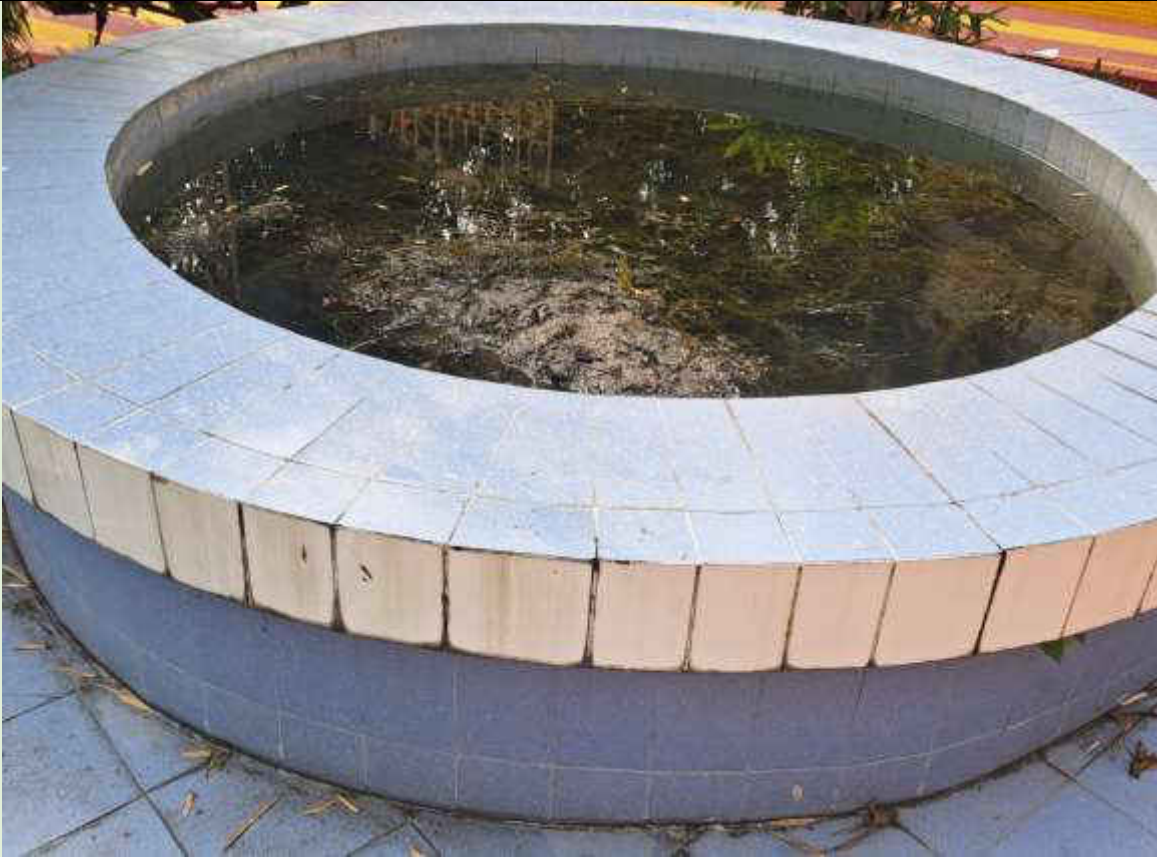
Rain water storage
