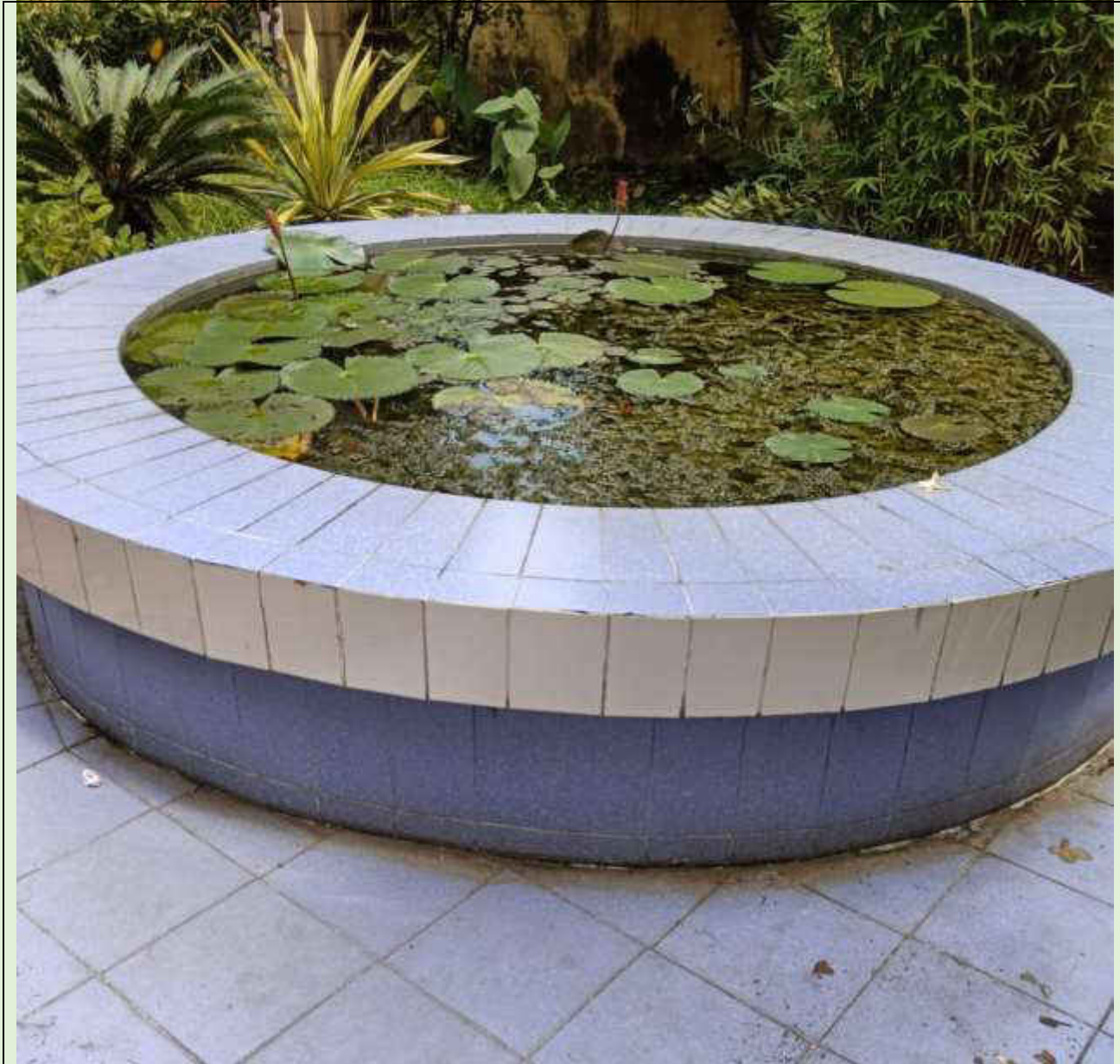
Water lily plantation in Rain water storage
